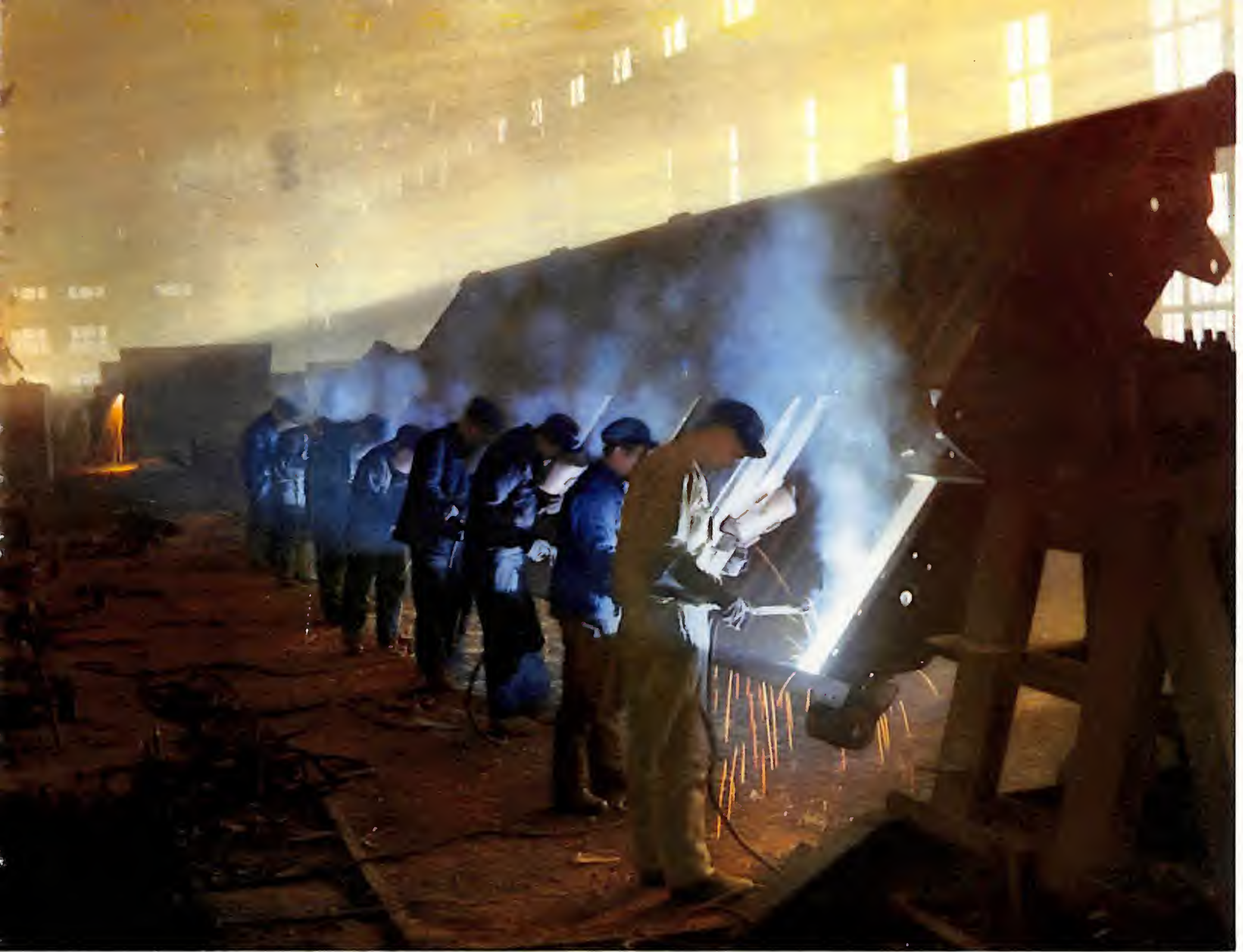
Electric welding on the bottom of a mine tip-car.
